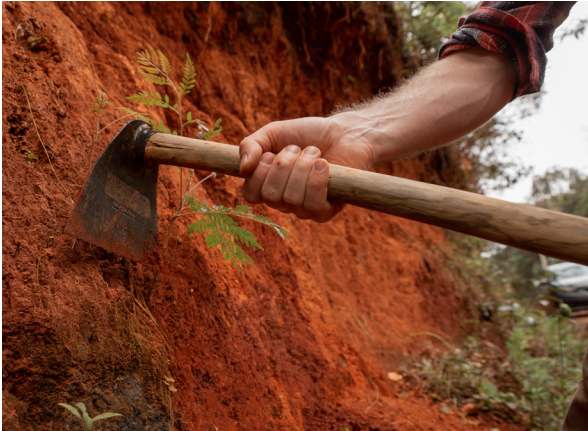
STEP 1. Superficially clean the ravine.
