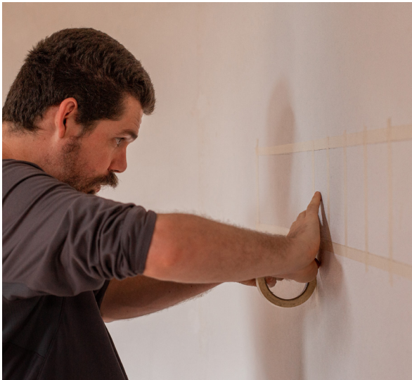
STEP 2. Use adhesive tape to define the spaces for the application of each sample. Suggestion: mark 10 by 15cm rectangular spaces for each sample/color.
